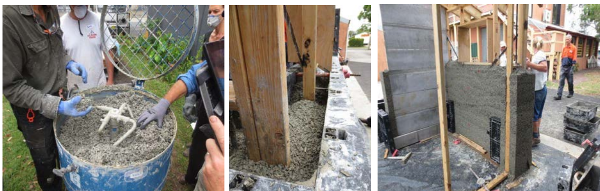
Figure 23: Mixing and tamping of hempcrete into a construction frame (Gregor, 2014)
