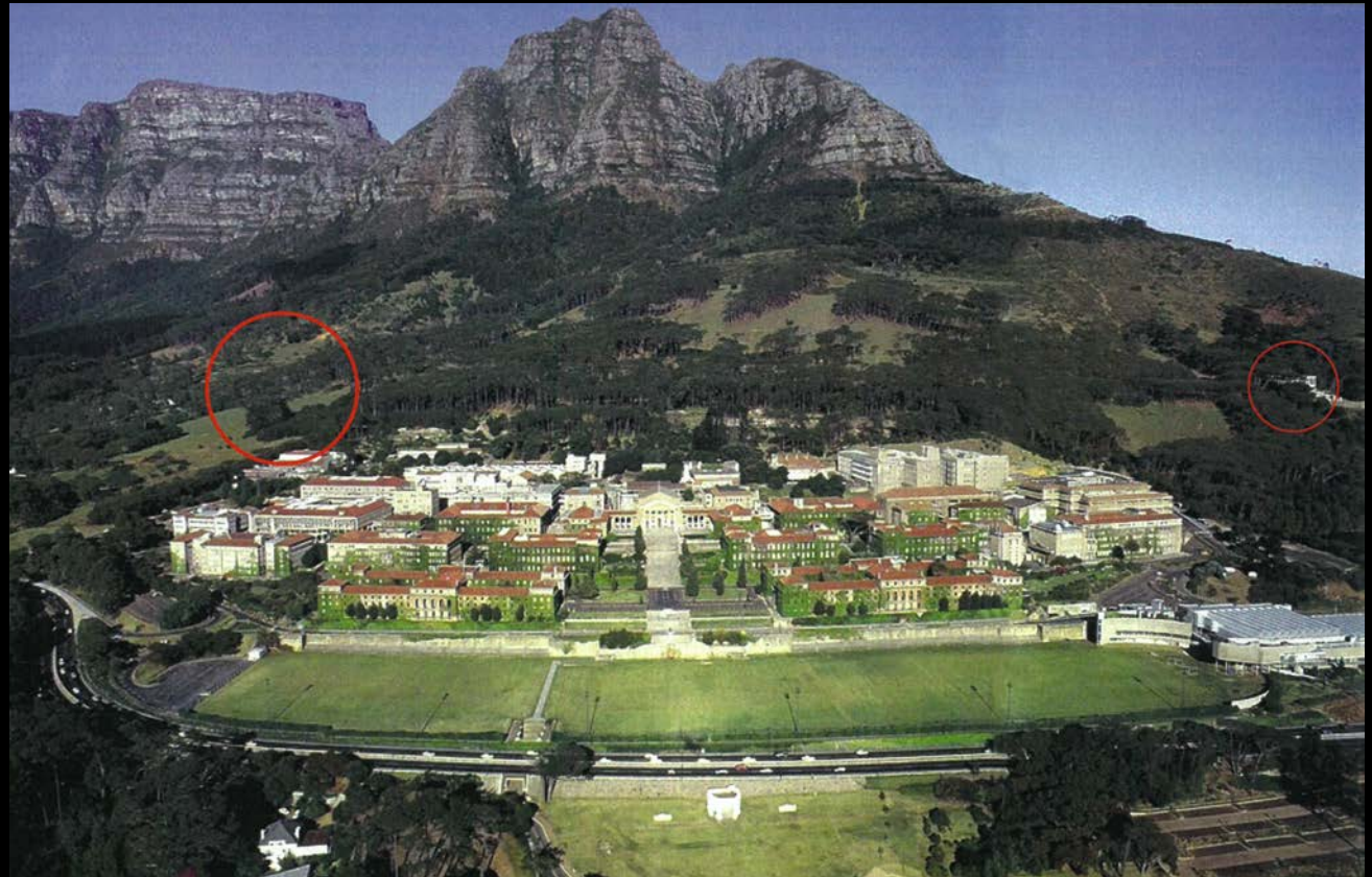
The left hand circle marks the proposed site of the Nelson Mandela School. The circle on the right marks the existing Rhodes Memorial.
